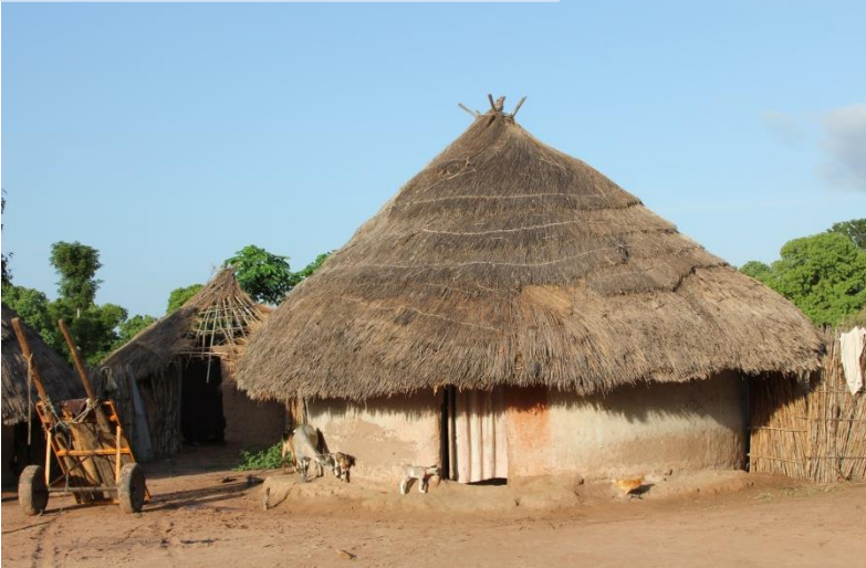
Poorly screened houses
