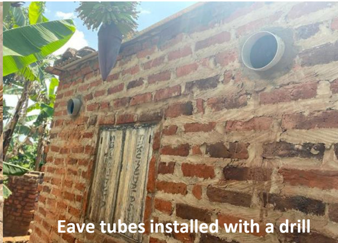
Eave tubes installed behind the vent
